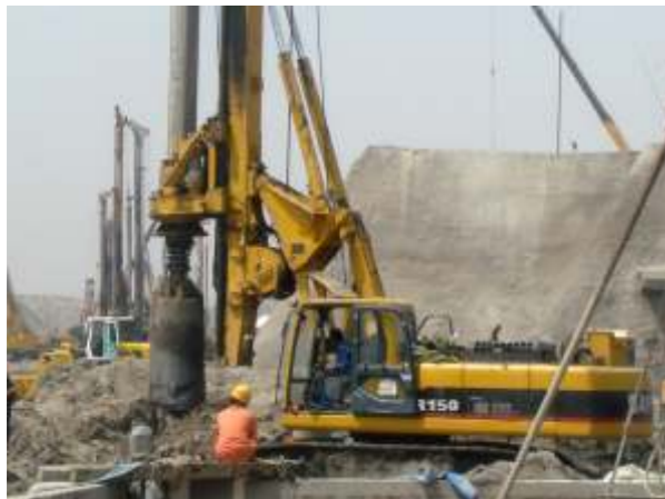
Zhengxi Railway passenger dedicated line project
