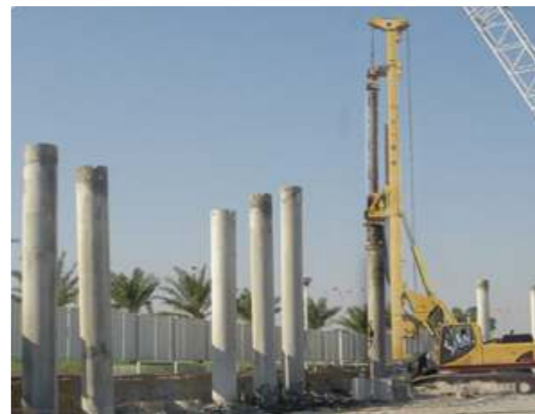
Airport construction in Doha, Qatar.
