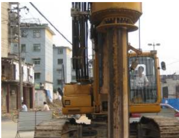
Xi'an urban construction site
