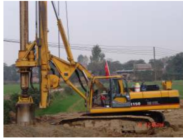
Wu Guang Railway construction site
