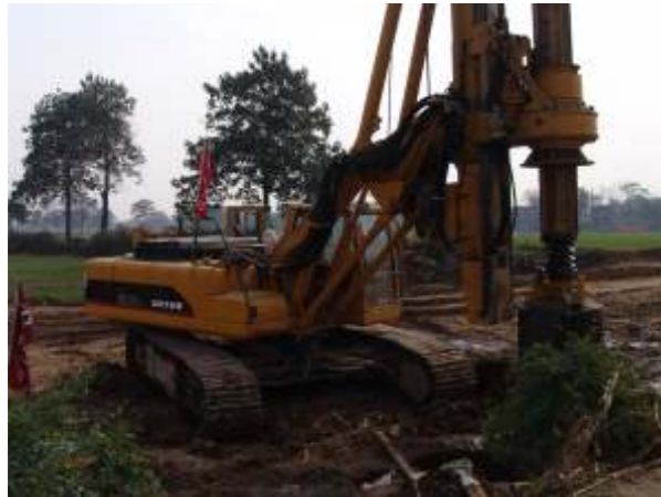
Yinchuan Yellow River Bridge construction project
