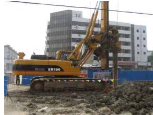
Hefei municipal construction site
